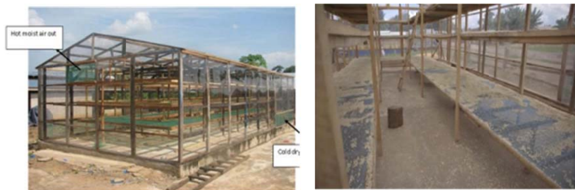
Figure 10: Large scale maize solar dryer by MoFA- inside and outside view
