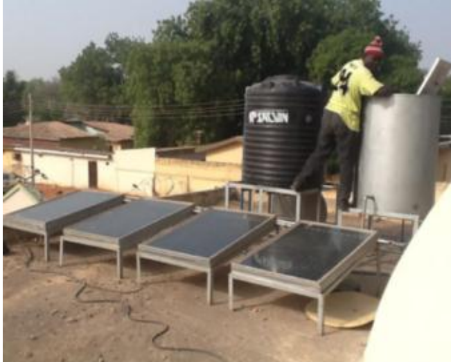
Figure 3: Locally made flat plate collectors by SERC UDUS
