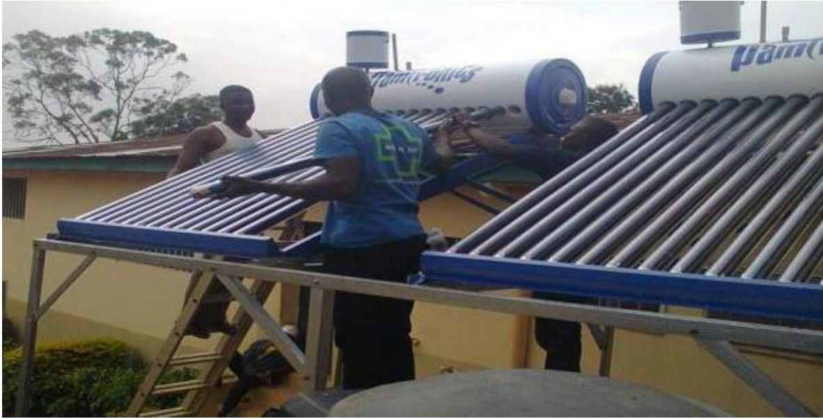
Figure 2: A typical solar water heating system.
