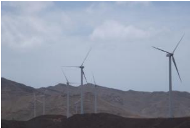
6 MW Wind Farm, in Sao Vicente, Cape Verde Commissioned November, 2011
