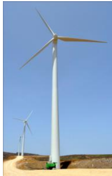
8 MW Wind Farm, in Sal, Cape Verde
