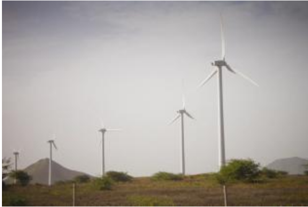
10 MW Wind Farm, in Santiago, Cape Verde Commissioned November, 2011
