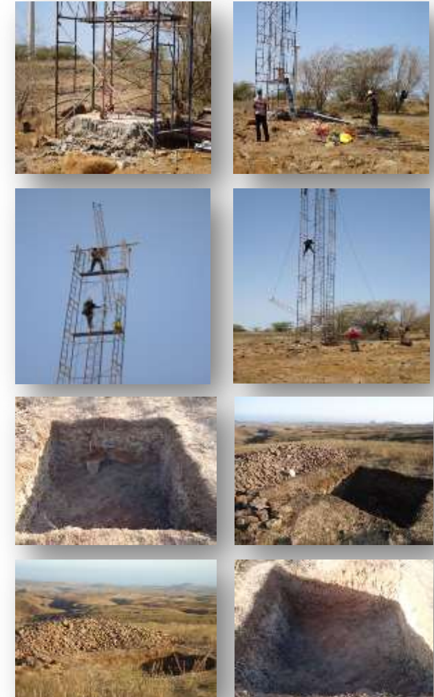
Meteorological mast erection works
