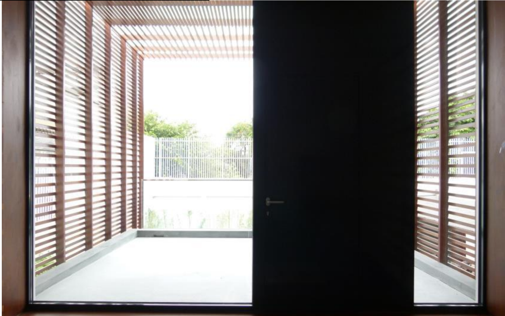
Austrian Embassy Jakarta: two-pane thermal glazing U-Value: <1,1\text{W/m}^2\text{K} , g-Value 0,3
