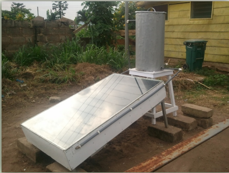
Solar water heater
