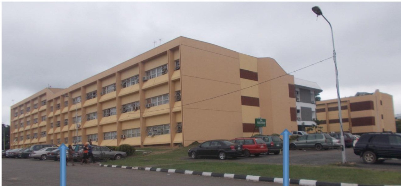
Eastern side of the building
