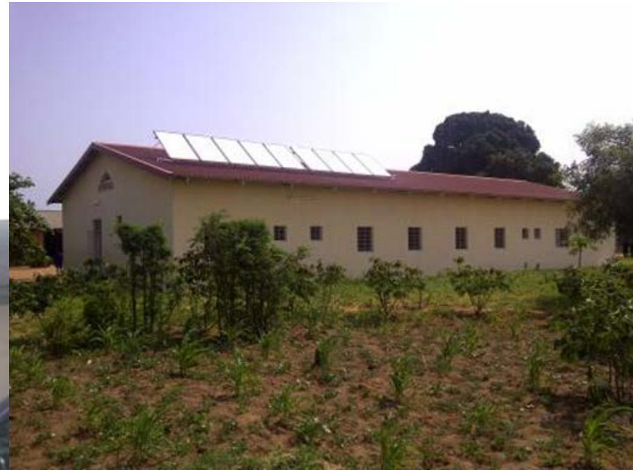
Ndlavela Hospital, Maputo, Mozambique
